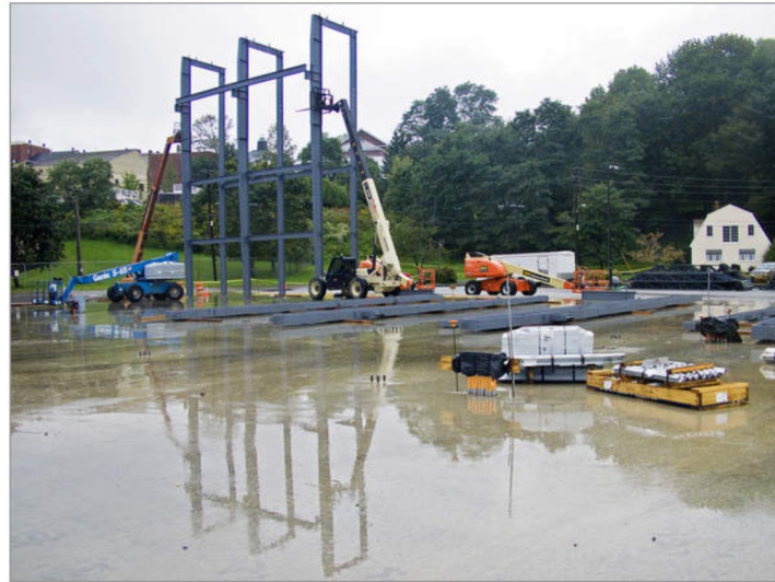
Maine Coast Construction erects the first steel girders of a new 55-foot tall, 22,000-square-foot boat repair shop at Front Street Shipyard, Sept. 16. Current plans show the shipyard moving into the building before Thanksgiving.
